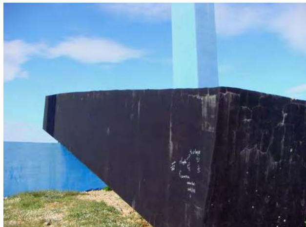
**Figure 5** Detail of a work by Tano Festa, showing damage to the black latex paint on concrete from light exposure, rain, and graffiti. Tano Festa, *Monumento per un Poeta Morto*, 1989 (detail). Situated in Fiumara d'Arte, Sicily. Courtesy Fondazione Fiumara d'Arte. Photo: Tom Learner.
