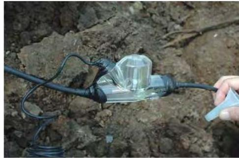
**Figure 10b** Plastic housing is used as a cable connection.
