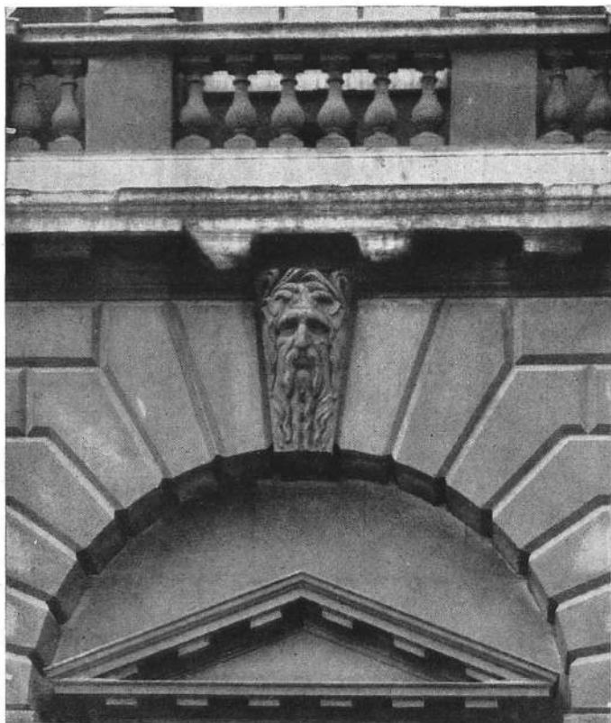
Fig. 12. Keystone, Strand Front, Somerset House, London.
