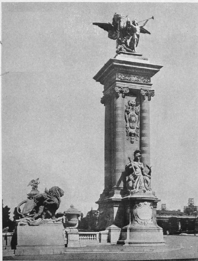
Fig. 38. Pylon to the Alexandre III Bridge, Paris.
