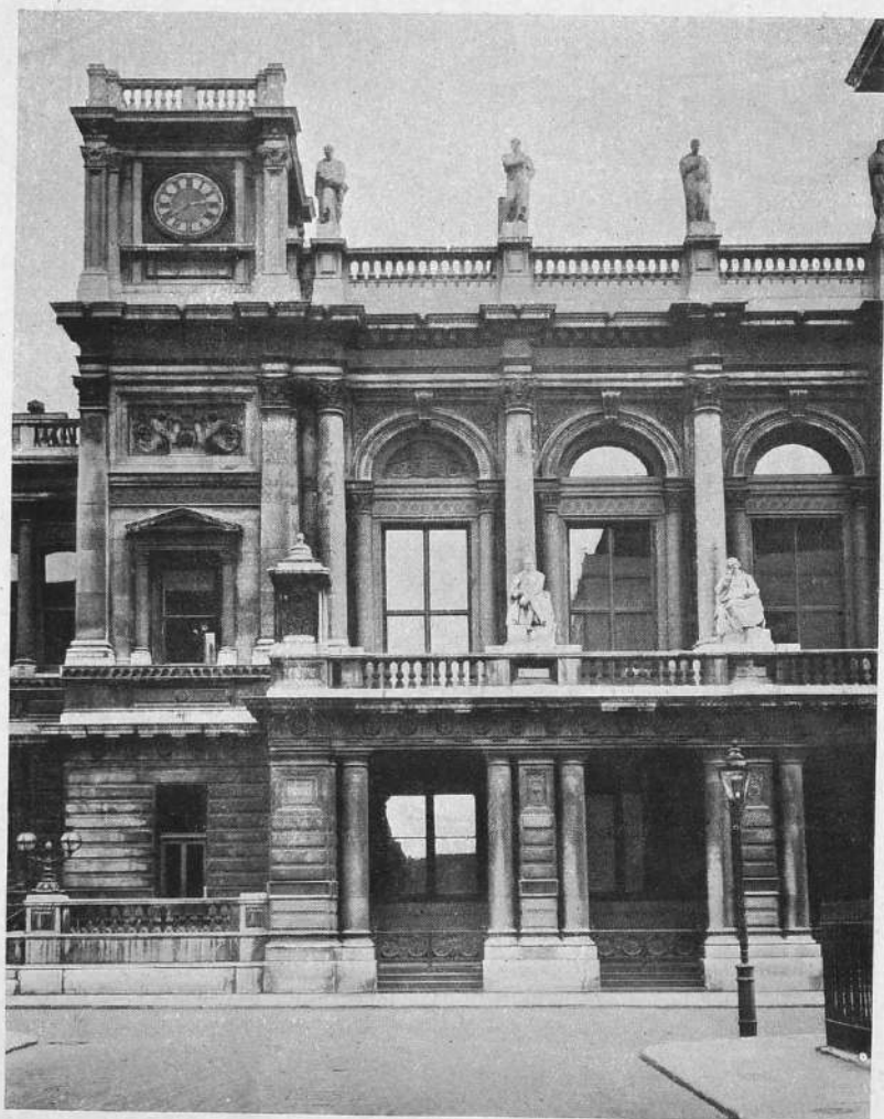
Fig. 28. The Civil Service Commission, Burlington Gardens, London.
