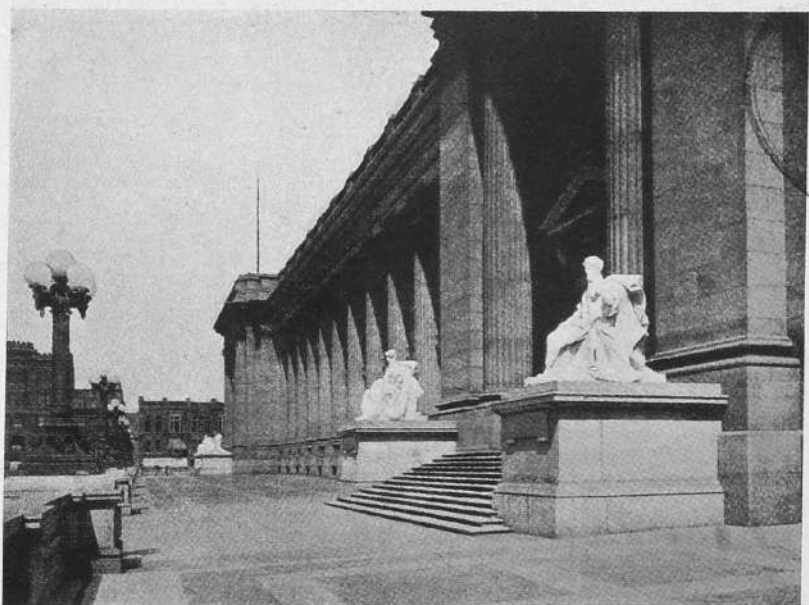
Fig. 37. Federal Court House and Post Office, Indianapolis.
