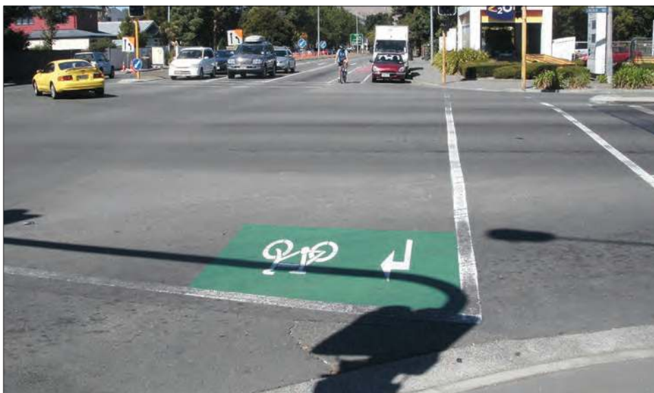
Figure 12.4: A hook turn box to allow two-stage right turns, in Christchurch, New Zealand. (Source: Author.)
