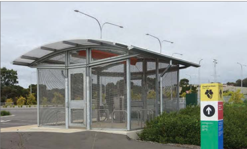
Figure 16.19: Australian Standard Class 2 communal locked cage. (Source: author's own work.)
