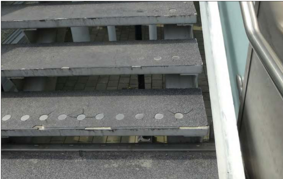
Figure 16.11: A simple wheel ramp installed alongside steps. (Source: author's own work.)
