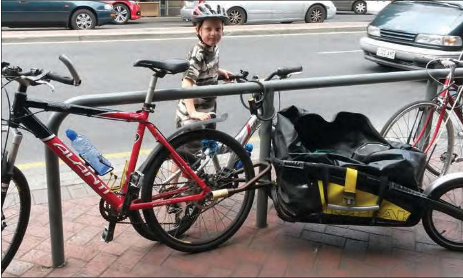
Figure 16.16: Long rail accommodates larger bicycles and trailers. (Source: author's own work.)
