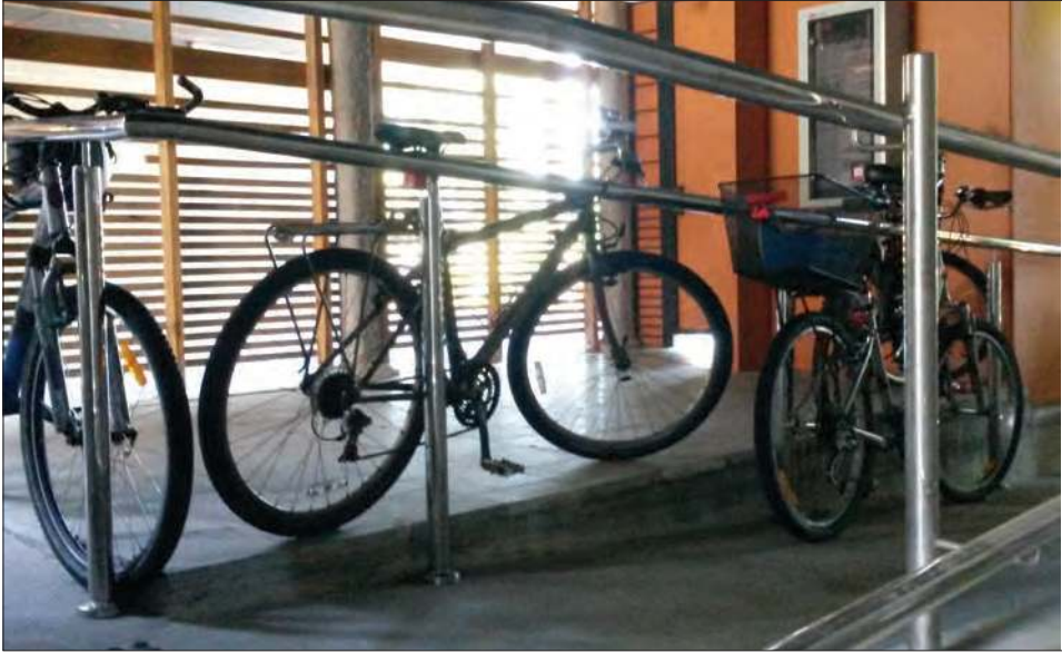
Figure 16.6: Bicycles stored on a disability access ramp at affordable housing apartments, Adelaide. (Source: author's own work.)
