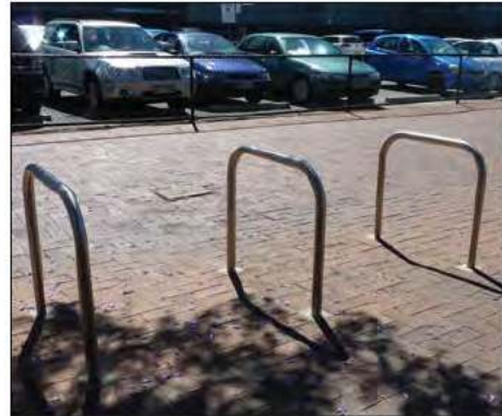
Figure 16.21: 'Flat top' rails stacked, with room for two bicycles with panniers at each rail. (Source: author's own work.)
