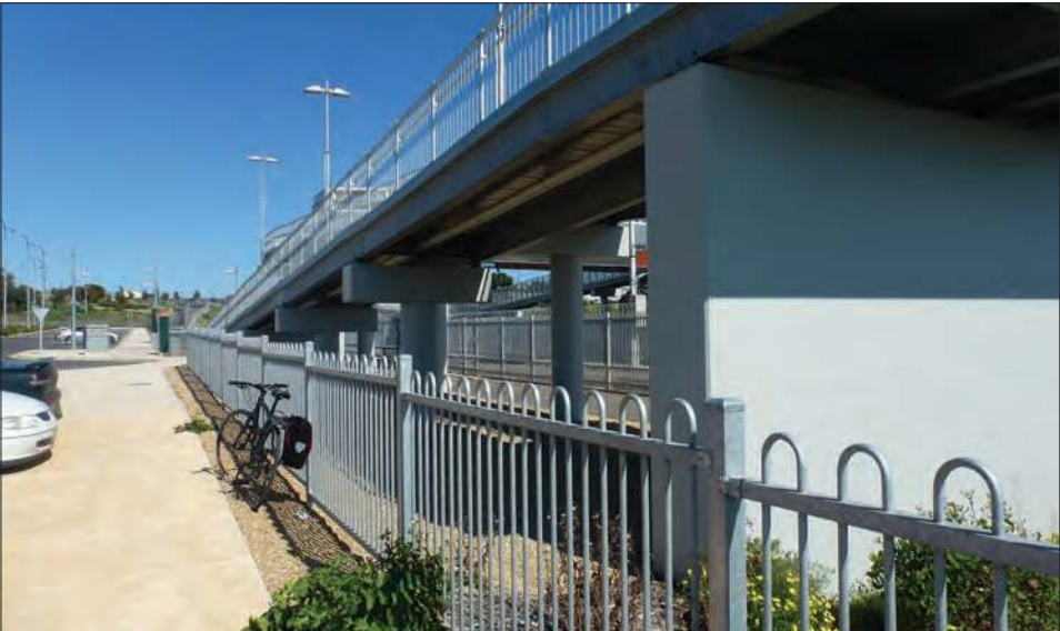
Figure 15.23: Safer alternatives for the bicycle cage at Seaford Meadows Station. (Source: Author's own work.)
