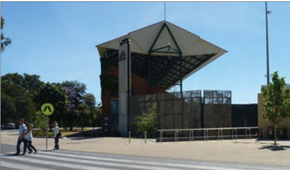
Figure 16.37: Long stretches of kerb ramp help reduce pedestrian and cyclist conflict. (Source: author's own work.)
